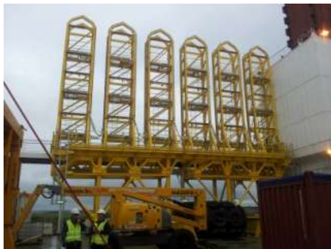
圖 61 Seafastenings for blade above the deck
